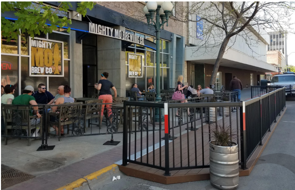
Great Falls' "pedlet" approach to maintaining a clear path of circulation and accommodating cafe seating.
