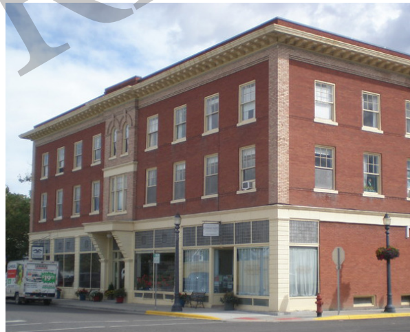
The restored Grabow Hotel, provides high-quality, upper floor lodging to visitors of the Downtown.
