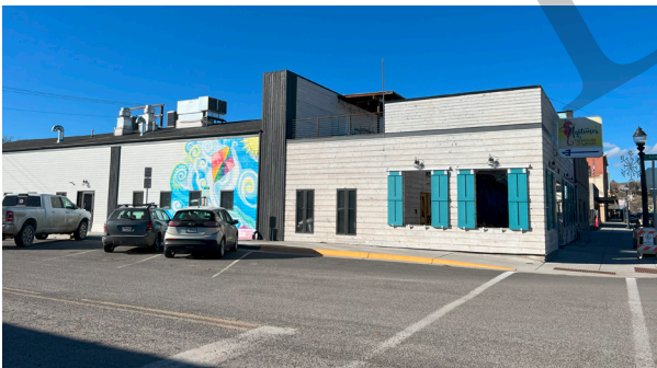
Angled parking in select locations along east-west streets, such as what exists on Clark Street, can help to subtly increase parking capacity in the Downtown.
