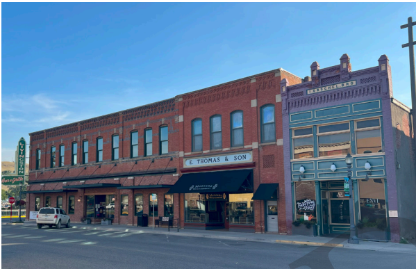
Active Ground Floor Uses
