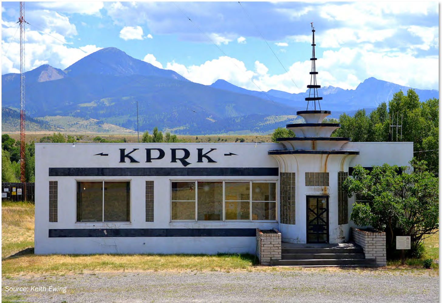
Figure 2.8: KPRK Radio Station
