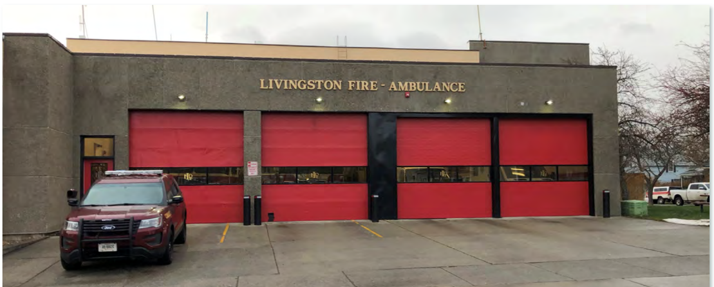
Figure 7.2: Livingston Fire Station
