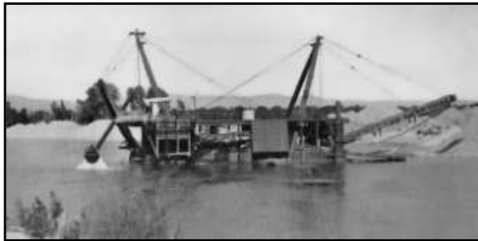
Photo 64. Historic dredging operation. Photo source unknown.
